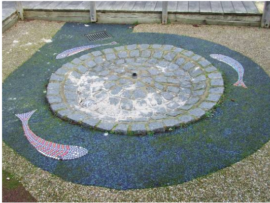
Image 2: A water feature that is accessible to all users but not working due to technical difficulty.
