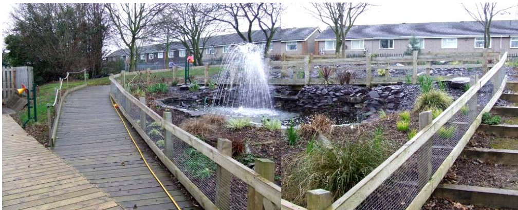
Image 5: This ramp is hardly used due to its slippery surface, especially when damp while the stairs are inaccessible to wheelchair users. Consequently, users use another route for access.
